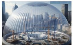
strength, weather-resistant materials and is supported by a continuous air pressure system, ensuring stability and safety throughout the construction process.
